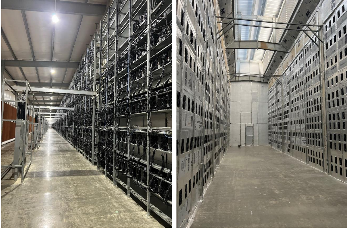
Source: Global X Research – The left graphic shows a single row of ASICs in a fan-cooled facility; this alley acts as a wind tunnel as each ASIC pulls air through it. The right graphic shows what's behind the wall in the left graphic. Hot air is exhausted into an insulated heat aisle before exiting the building.
